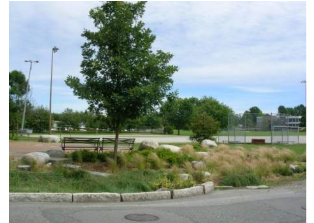
Inspecting Constructed Best Management Practices (BMPs)
