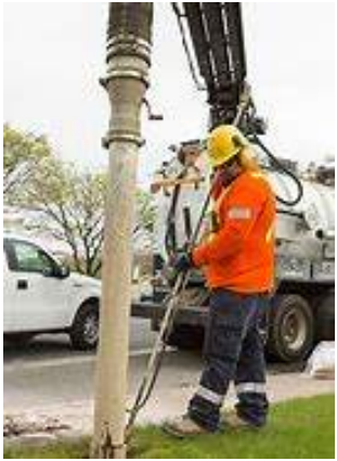
Catch Basin Inspection and Cleaning
