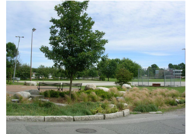
Inspecting Constructed Best Management Practices (BMPs)
