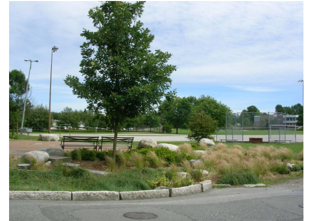
Inspecting Constructed Best Management Practices (BMPs)
