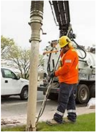
Catch Basin Inspection and Cleaning
